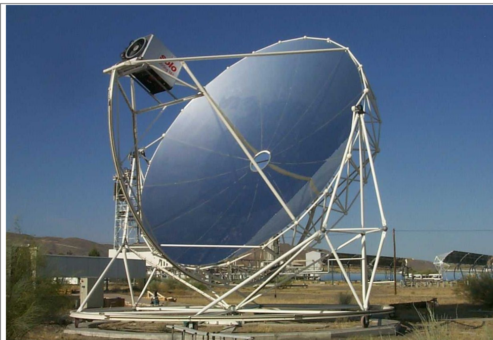
Figure 1 : Point focus parabolic mirror with Stirling engine at its centre and its solar tracker at Plataforma Solar de Almería (PSA) in Spain
