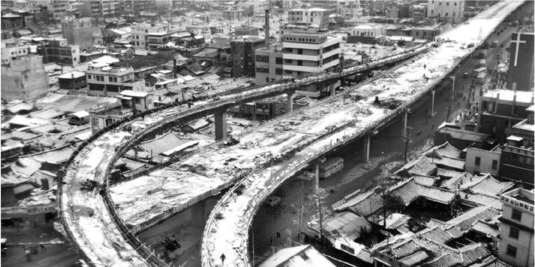
Cheonggyecheon motorway under construction in 1975
