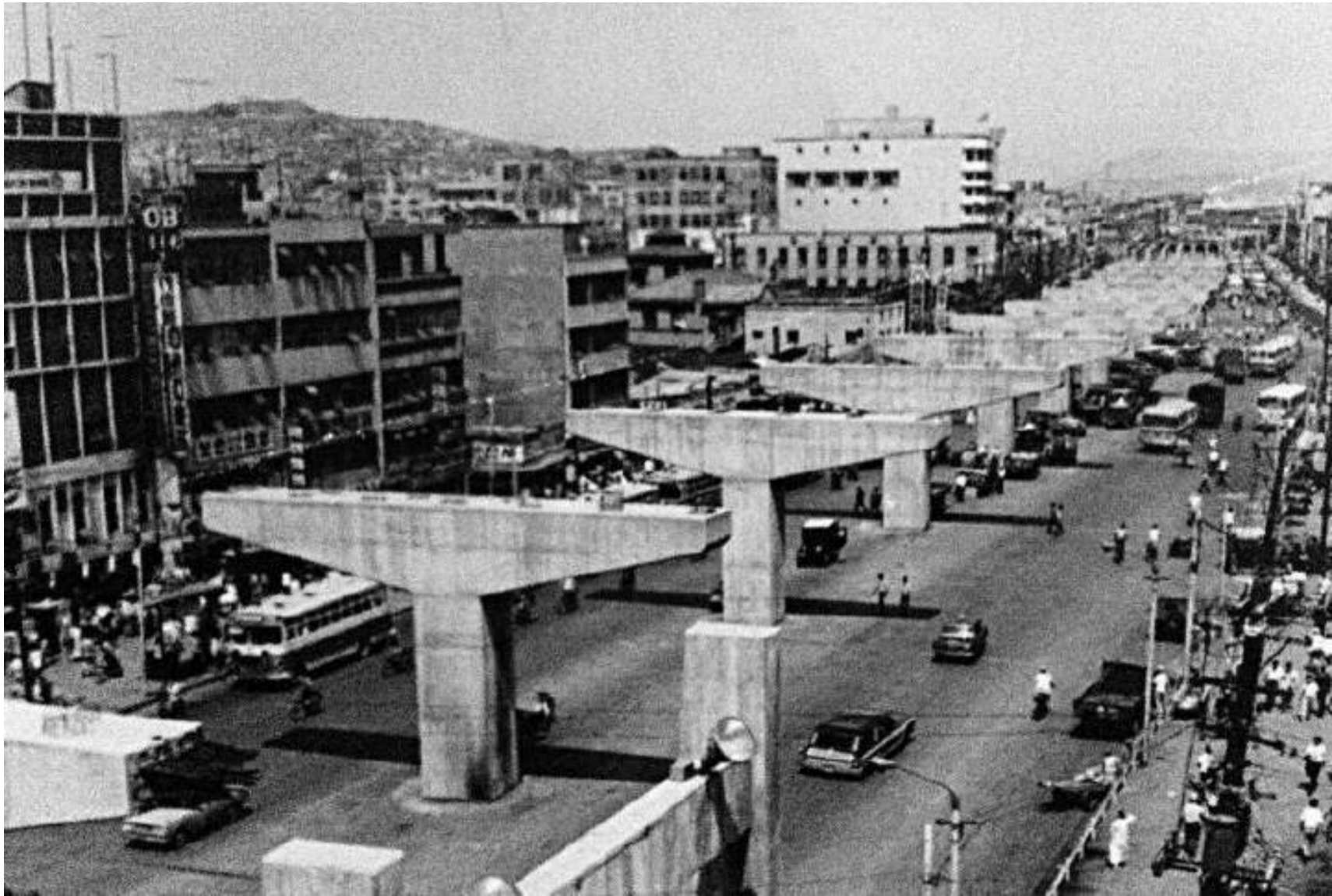
Cheonggyecheon viaduct under construction en 1970
