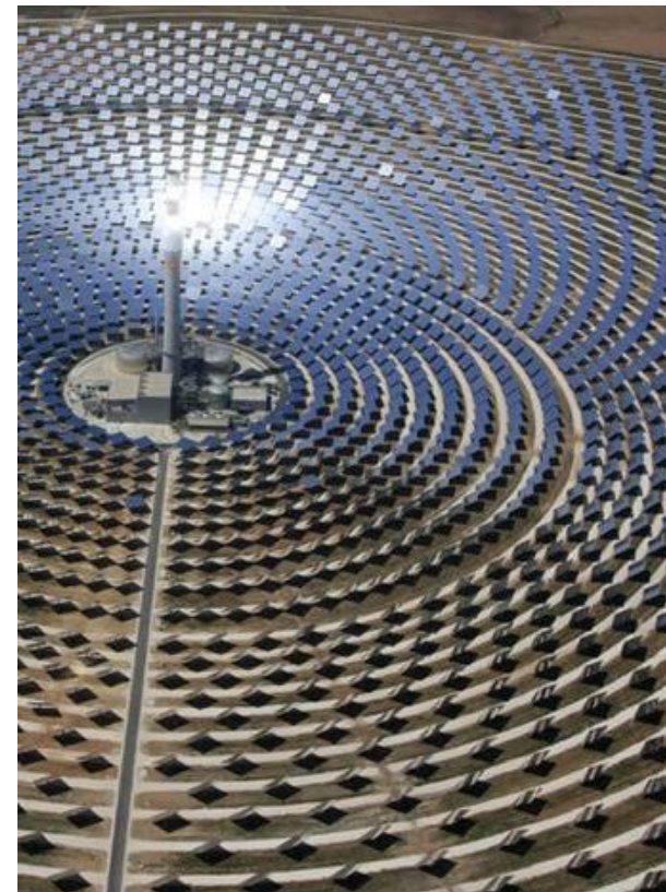
To heat then electricity Concentrated Solar Power(CSP) 20% efficiency
